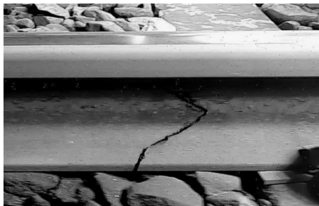
Output: Railway Track Crack Detected
